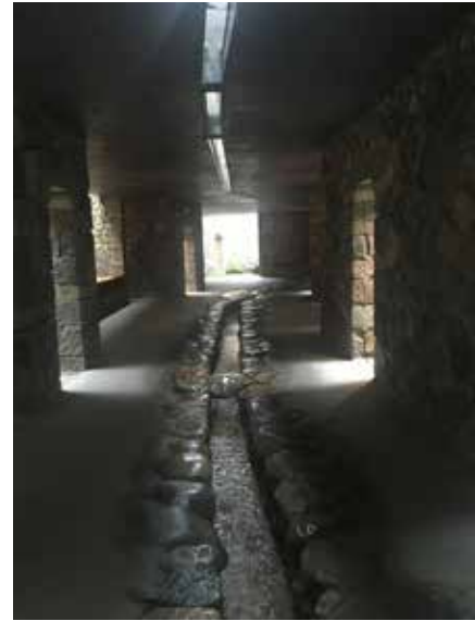
6. Top light as spatial approach as with the example of Shicang Indenture Museum ©Zhen Zhang
