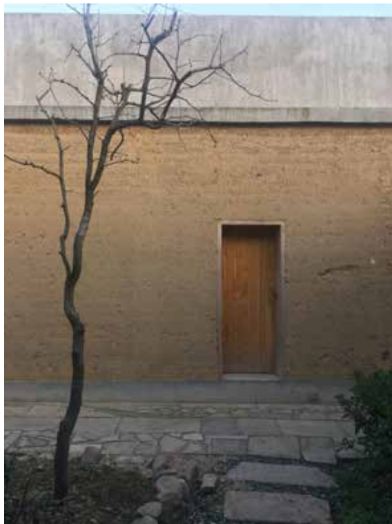
15. Concrete roof and rammed earth wall as a materiality approach seen in Wangjing Memorial Hall ©Zhen Zhang
